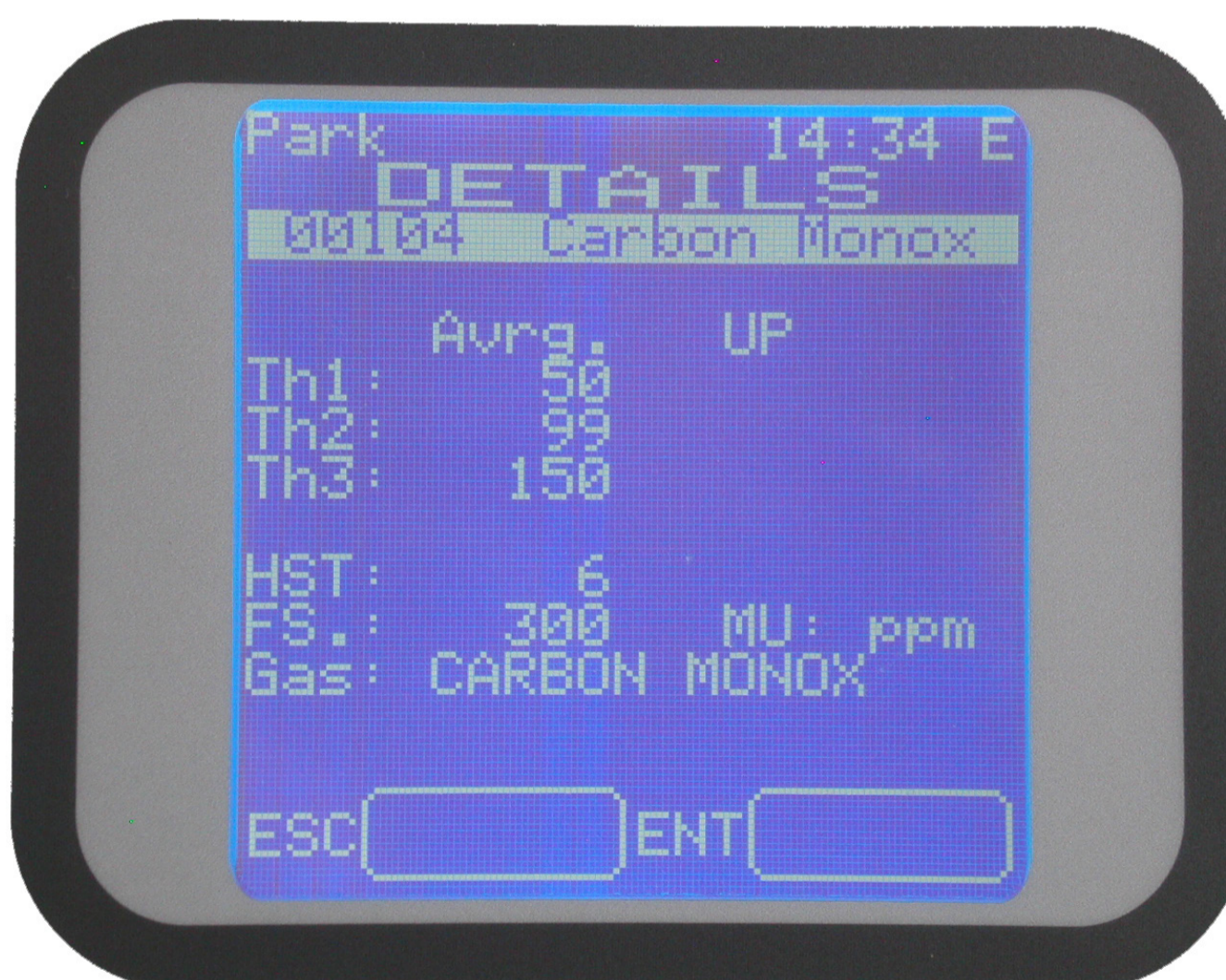
Figure 42 Detector details screen in "Engineer" level
